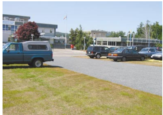
A permeable parking lot at the Vancouver Island Technology Park. PHOTO: Aqua-Tex Scientific Consulting Ltd.
